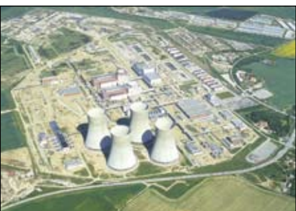
The 2000MW Temelin Power Station in the Czech Republic.
