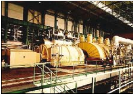
The machine hall of Dukovany Power Station in the Czech Republic, comprising eight 220MW combined cooled generators.
