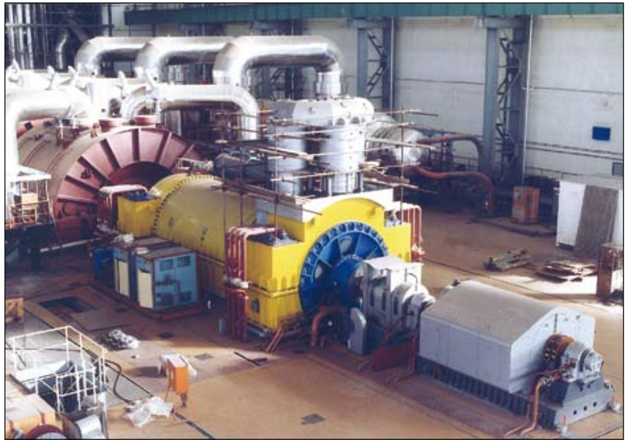
The machine hall of Dukovany Power Station in the Czech Republic, comprising eight 220MW combined cooled generators.
