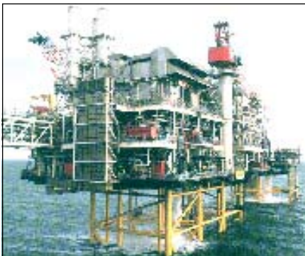
Ekofisk oil platform incorporating two BRUSH 25MW turbogenerators.
