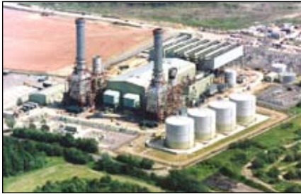
Corby power station utilising BRUSH DAX turbogenerators.
