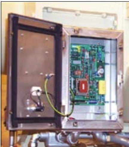
Fig.2 Receiver in IP66 enclosure for generator mounting
