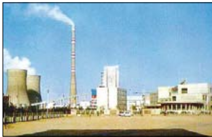
Shen Tou Power Station, Peoples' Republic of China.
