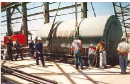
Installing the generator stator at Mejillones Power Station in Chile.
